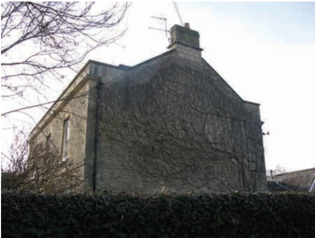
The Mansard roof at Exeter House
