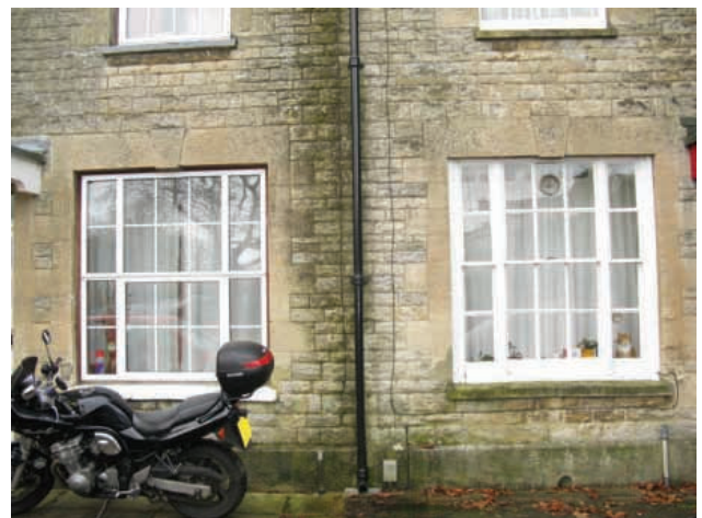
Replacement and original windows at 22 and 20 School Road respectively
