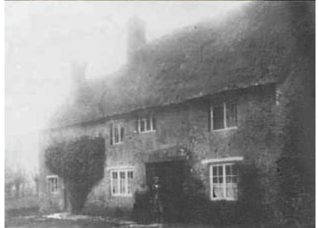
The Miller's House c.1910: a wall now divides the garden from the front and has a later extension © J. Kennedy
