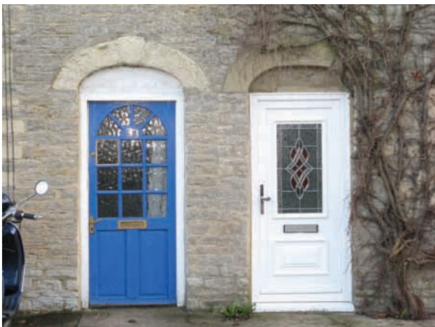
Modern doors and windows can be replaced to enhance the properties and return their original charm
