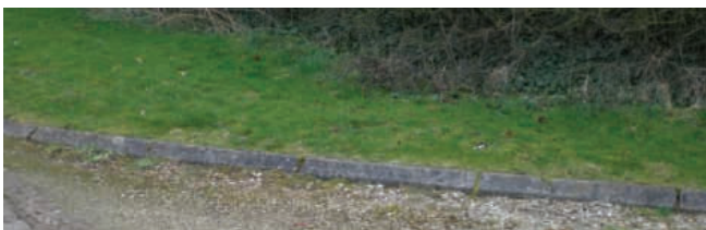
Concrete kerbs outside the electricity substation
