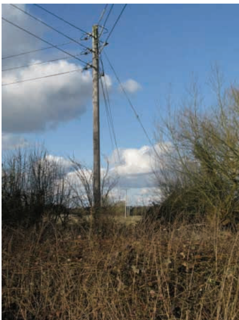
Telegraph poles marching across the land can be detrimental to the conservation area: careful negotiation is required to prevent this
