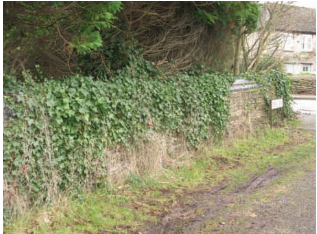
Rural verges can help to retain character while not providing any harm to modern vehicular accesses
