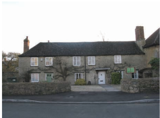
The former workhouse, 14 School Road
