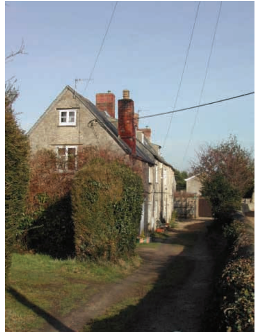
Cables continue to mar views of historic buildings
