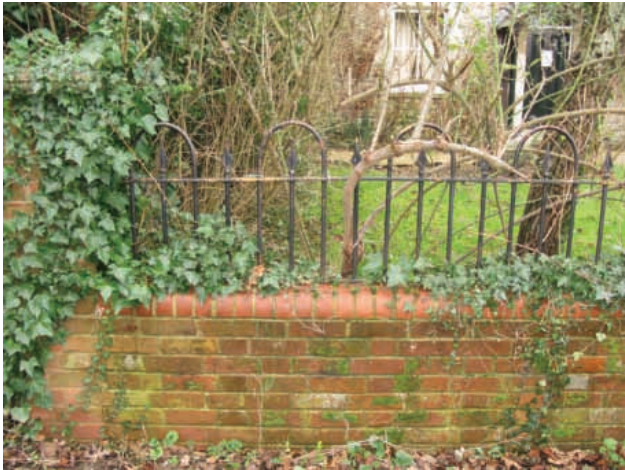
Wall and railings at 28 School Road
