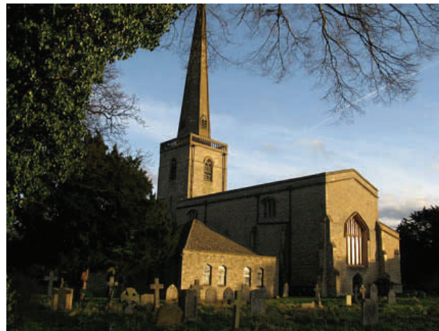
Church of St Mary viewed from the northwest
