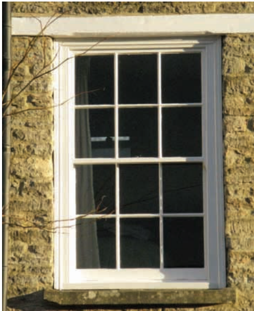
Modern materials which are sympathetic to the buildings are sometimes acceptable
