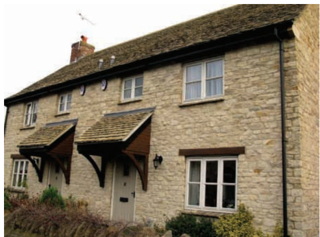
6-8 Church Street: natural stone and vernacular detailing encourages mitigation
