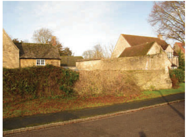
The high wall behind no.47 Mill Street
