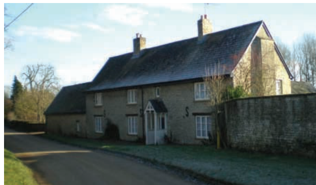
College Farm, vernacular style and limestone construction
