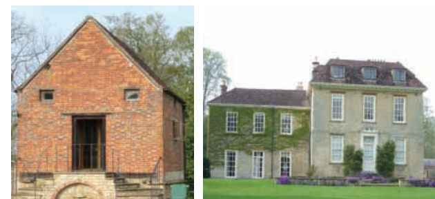
The Granary of Cottisford House & Cottisford House
