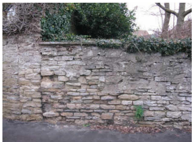
Traditional materials should be used to repair boundary walls
