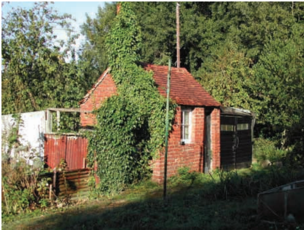
Brick outhouse: possible washhouse?
