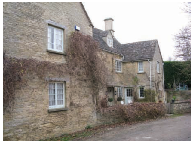
Mill House with its boundary wall and projecting gable
