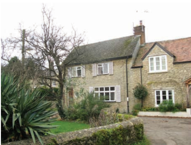
The tightly knit carriageway can cause parking difficulties which threaten the tranquillity of the area
