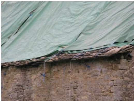
Roof tiles failing at Grade II Listed Mill House Barn: December 2008 (above and below)
