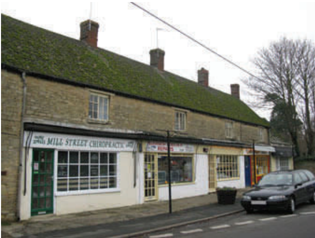
Mill Street Shops
