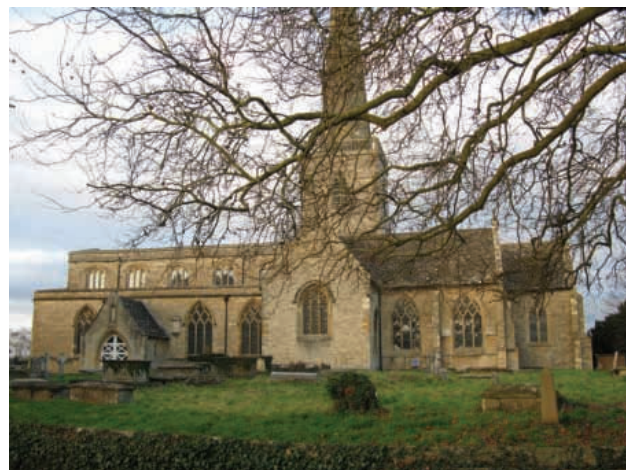
The Church viewed from the south
