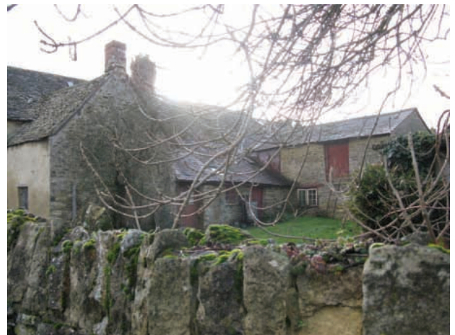
The outbuildings of 115 High Street
