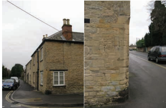
The strong building line and chamfered corner at 2 School Road
