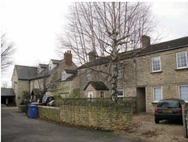
Nos. 52-56 Crown Road
