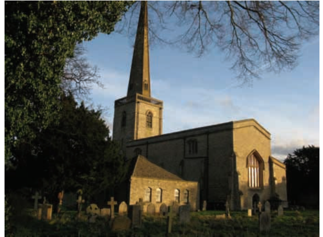
The west elevation of the church
