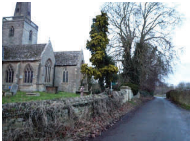
Limestone boundary wall at the church
