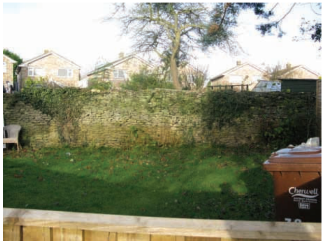
Boundary wall to side of no. 36
