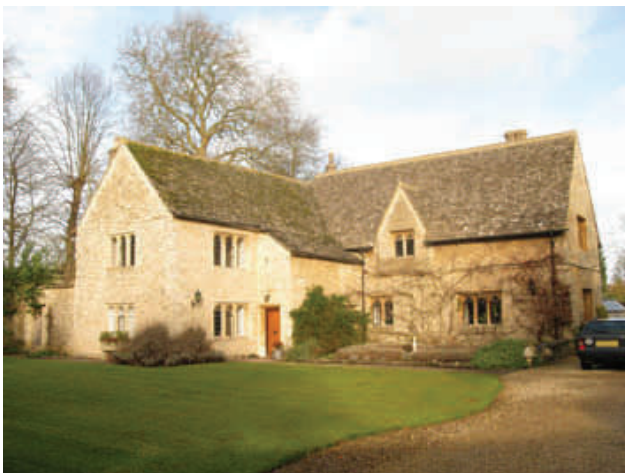
The Old Vicarage, 39 Mill Street
