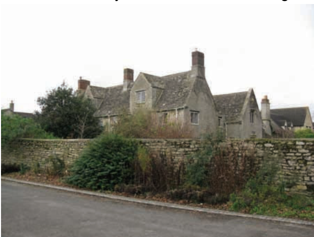
No. 42—The Court House
