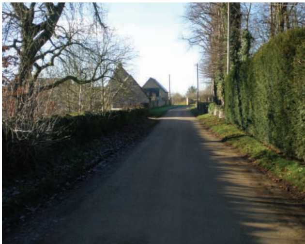
Erosion to grass verges looking east towards College Farm
