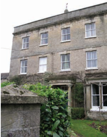
The classical parapet features of no. 101 High Street
